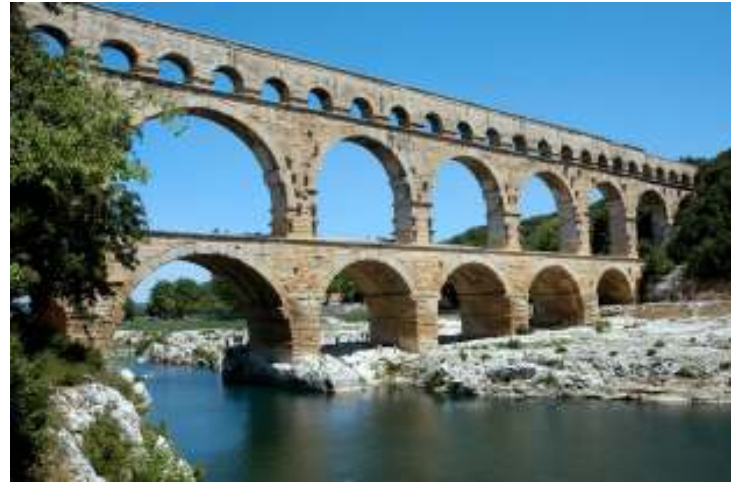
A Roman aqueduct that is still standing! lillisphotography/iStockphoto.com
